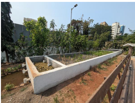
Source: Eco-STP(recycles sewage water of 42,000 litres/per day), Marol Urban Forest, WRI India
